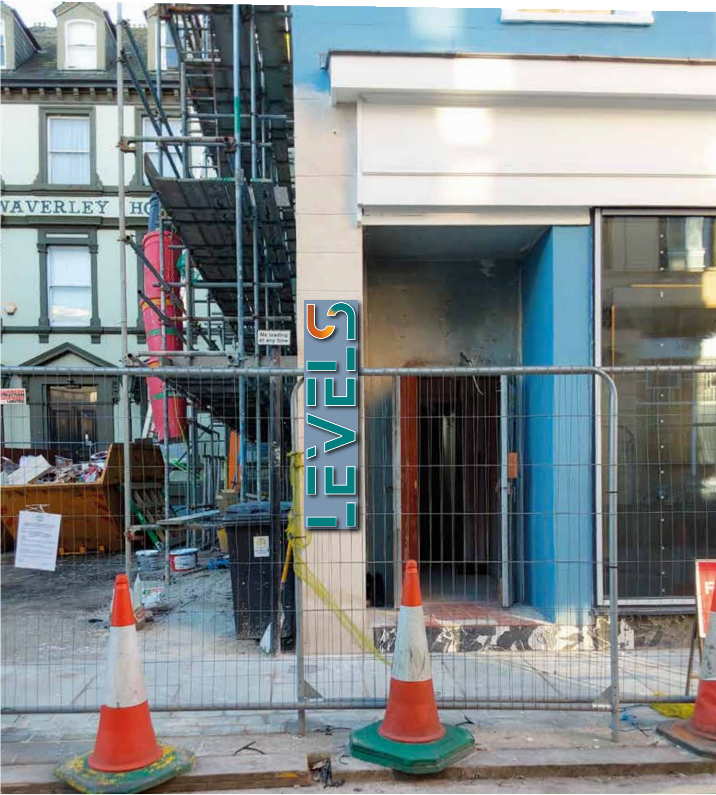
ITEM A 403mm (w) x 1850mm (h) Built up letters fitted onto signtray with 50mm returns 442mm (w) x 1890mm (h)
